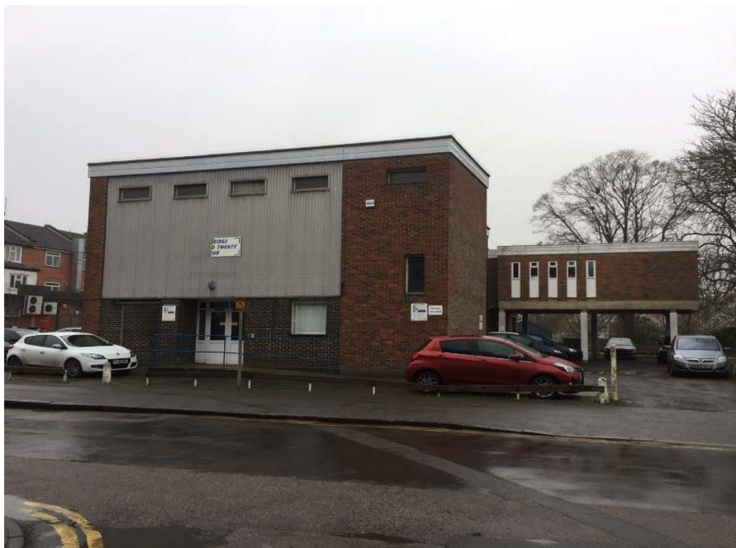
Teen & Twenty building looking west
